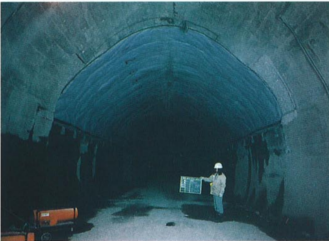
● PCL版据付前
