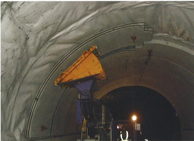
●PCL版据付前
