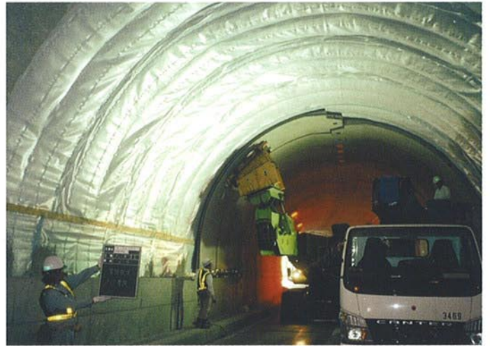
● PCL版据付状況-2
