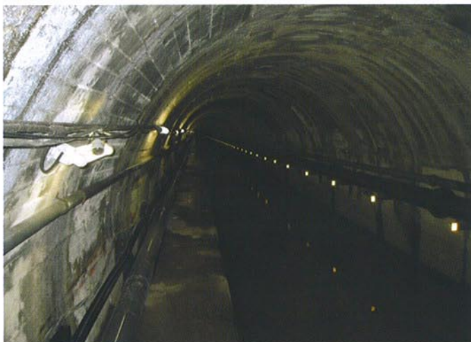
●PCL版据付前
